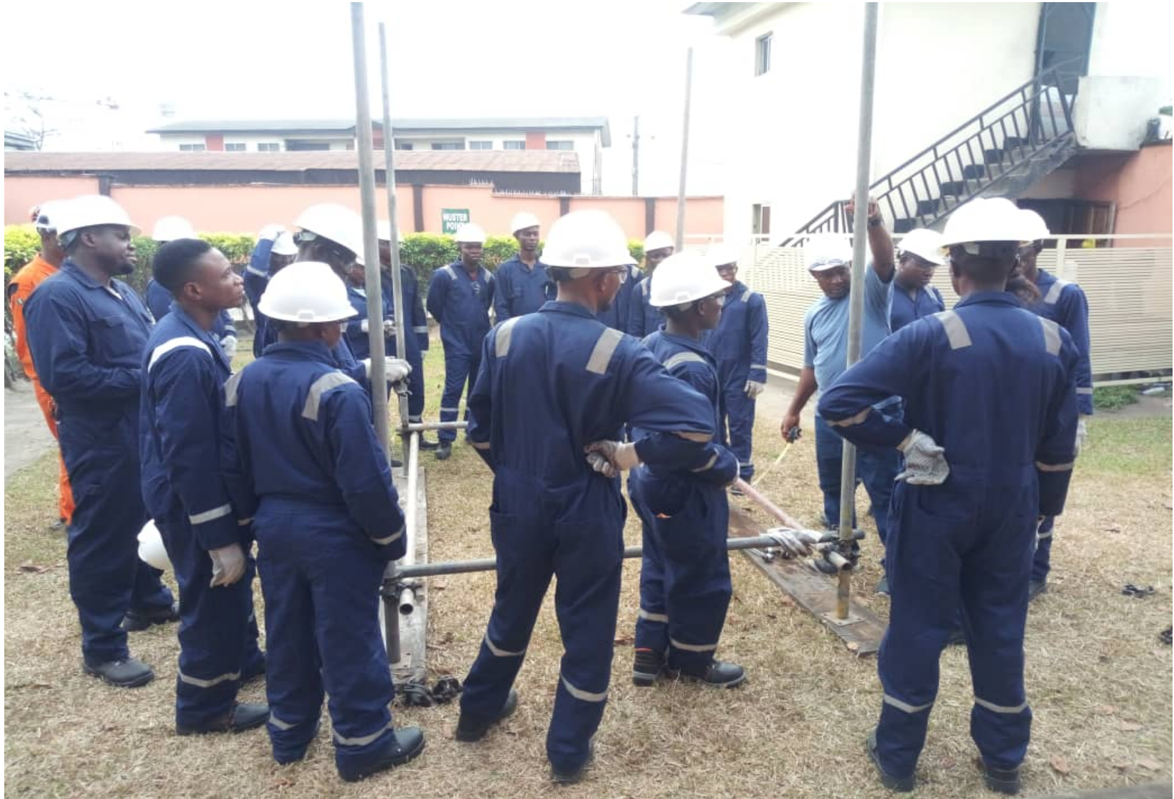
Picture 4: Trainees Erecting a Scaffold
